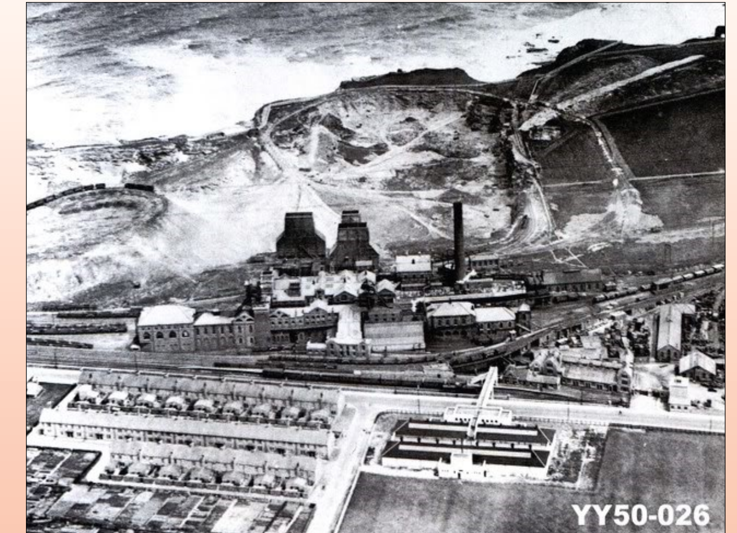
Whitburn Colliery, created to supply the lime kilns (date unknown) Photo Credit: Marsden Banner Group 2015
